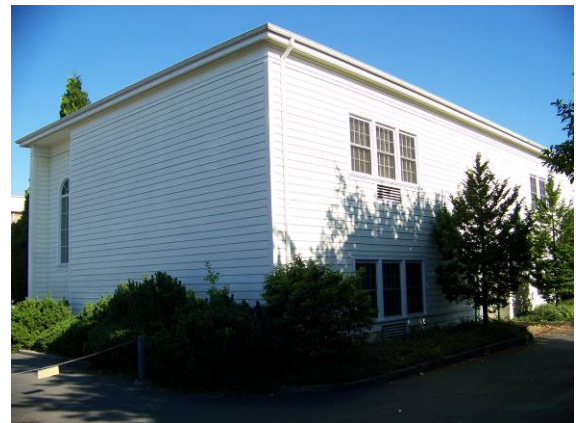
1992 Addition (230C), south and east elevations looking northwest.
