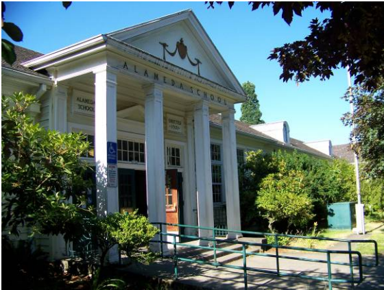
Main building (230A), north (front) elevation looking southwest.
