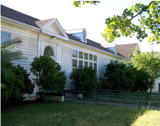
Main building (230A), west (side) elevation looking southward.
