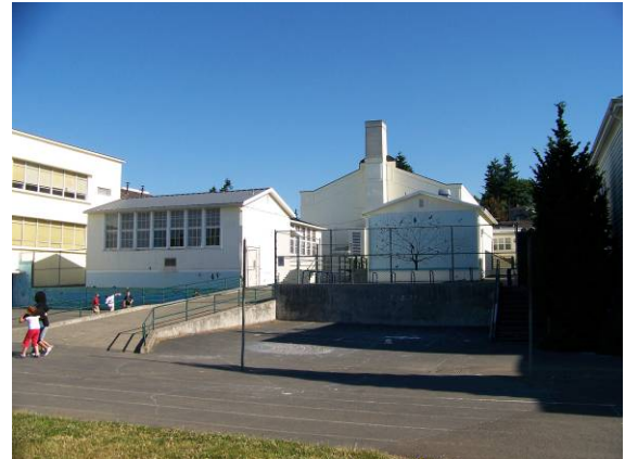
From left: 1954 Addition (230B), 1918 Portable Classrooms (230P2), Main building Auditorium (230A), and 1918 Portable Classroom (230P1), looking northward.
