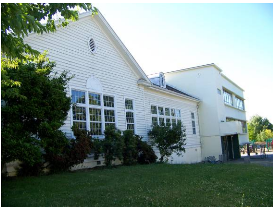
Main building (230A) and 1954 Addition (230B), west (side) elevation looking southward.
