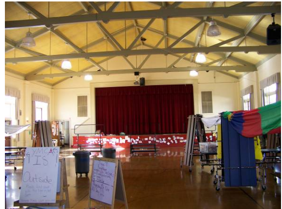
Main Building (230A), auditorium, looking south.
